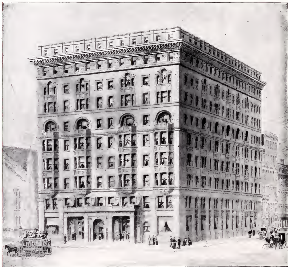
Holland House, New York. Heated and lighted by 448 H. P. of Babcock & Wilcox Boilers. Erected 1890.
